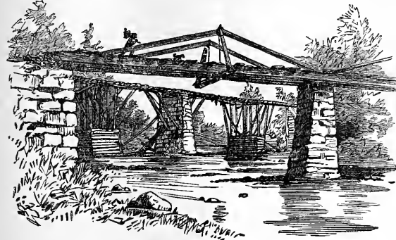
Bridge Across Platte Creek.
